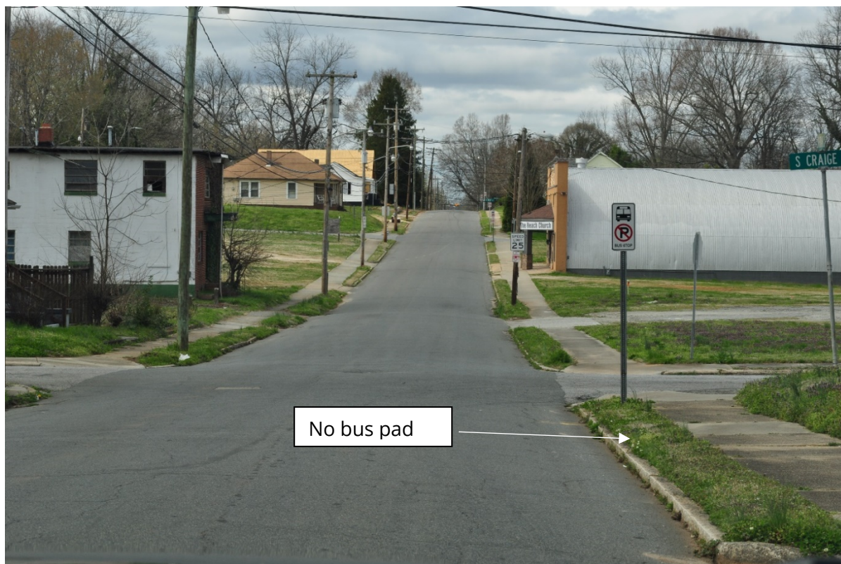
FIGURE 24: BUS STOP AND SIDEWALK CONDITIONS AT HORAH ST./CRAIGE ST. INTERSECTION
