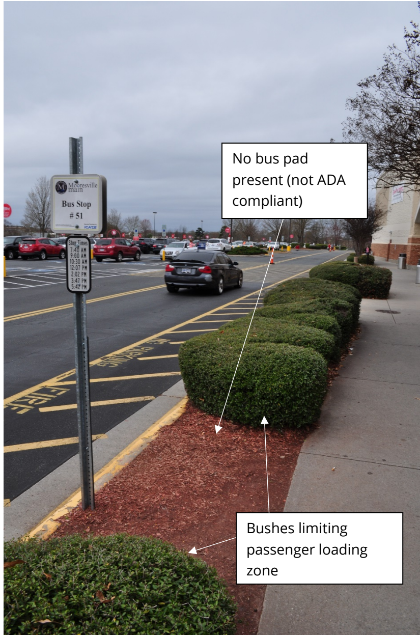
FIGURE 31: BUS STOP MISSING A BUS PAD AT MOORESEVILLE (EXIT 36)
