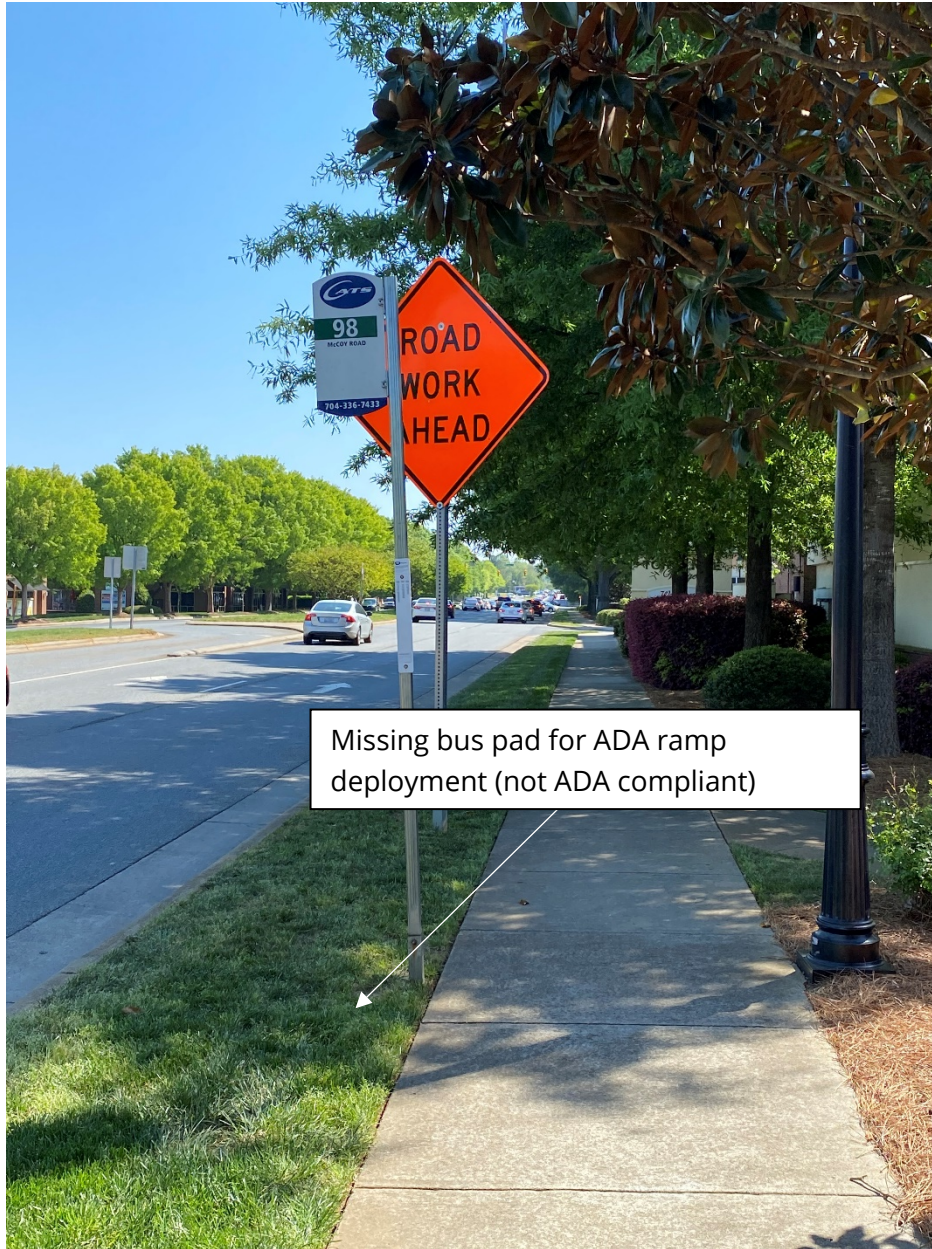
FIGURE 6: BUS STOP WITHOUT BUS PAD IN HUNTERSVILLE ALONG GILEAD ROAD
