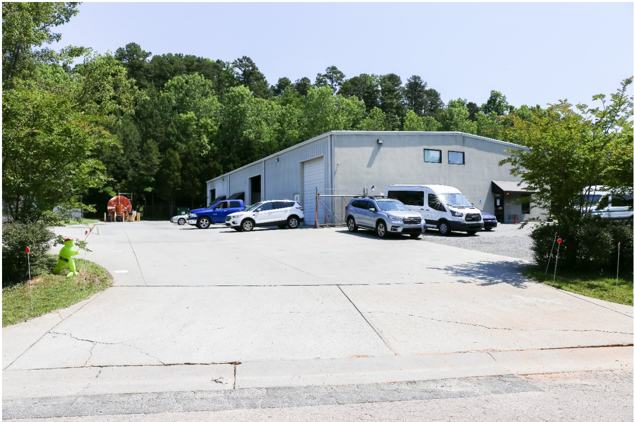
FIGURE 46: RIDER OPERATIONS AND MAINTENANCE FACILITY
