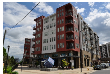
FIGURE 2 - TRANSIT IMPROVEMENTS IN CHARLOTTE HAVE SPURRED INVESTMENT IN TRANSIT SUPPORTIVE DEVELOPMENT
